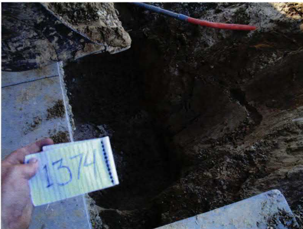
Picture 2: UST 1374Dove excavation pit.
